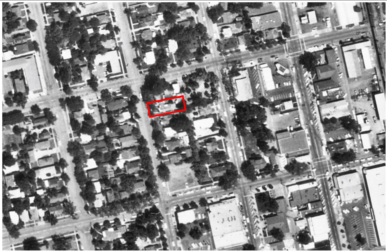
Source: UC Santa Barbara Library, Framefinder Aerial Imagery, CAS-65-130_14-213, 05/18/1965, accessed June 3, 2022.
